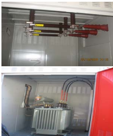
Compartment transformateur
